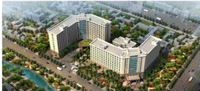
上海虹桥枢纽叶迪集团 Project in Shanghai Hongqiao
